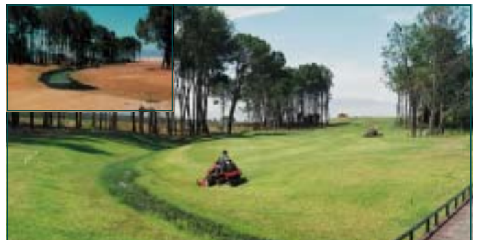
Figure 3 - MacMat channel (Inset : Immediately after construction)
