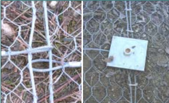
Figure 4 - Particulars of Steelgrid anchorage
