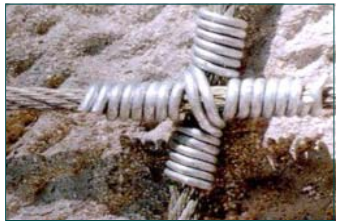
Figure 2 - Lacing node detail
